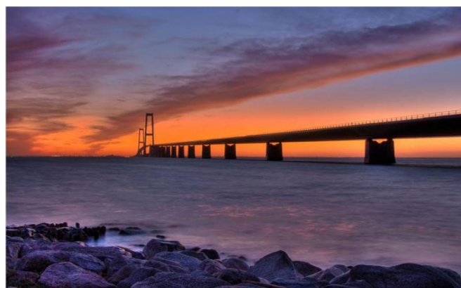
Figure 5: Denmark's great belt bridge
