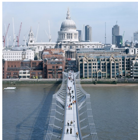
Figure 10: London's millennium bridge
